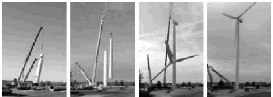
Construction of the school’s wind turbine
